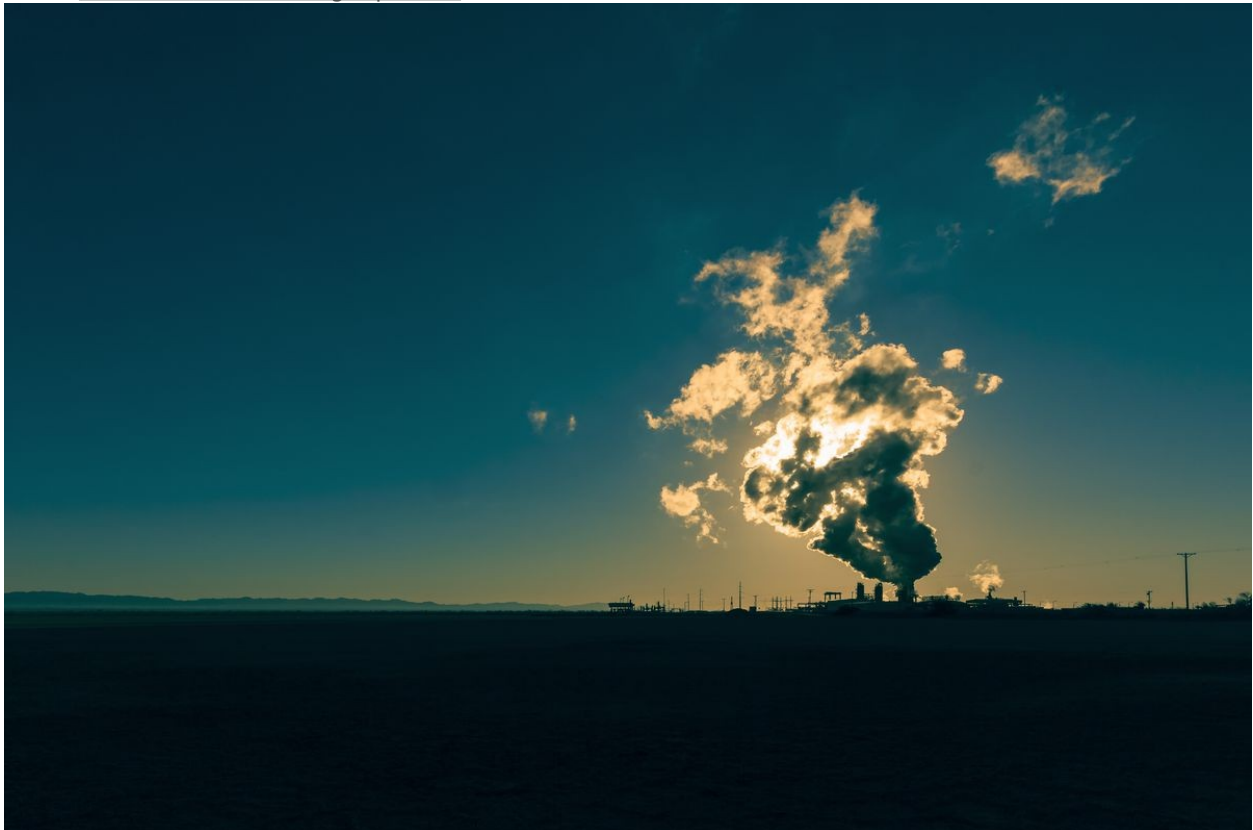
Sunlight glows through the steam of a geothermal power plant in Niland, California. Mickey Strider/Loop Images/Universal Images Group via Getty Images
