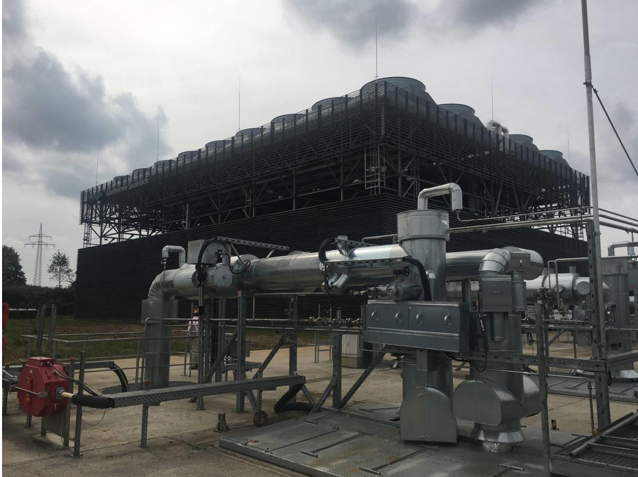
Sauerlach Geothermal Plant, a binary geothermal power plant in Munich, Germany. Tim Latimer
