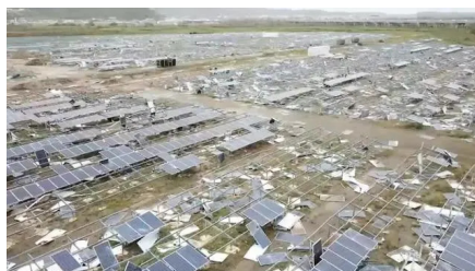
Figure 7.5: Damaged Puerto Rico solar plant
