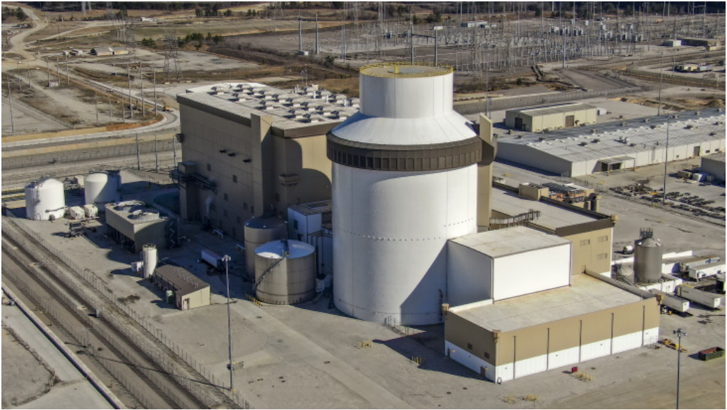
Alvin W. Vogtle Plant Unit 3, Georgia Power
